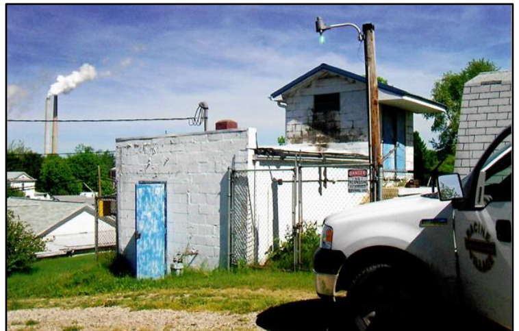
Old Water Treatment Plant, Village of Racine. Photo courtesy of the Village of Racine.
